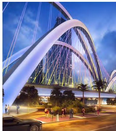
I-395 Bridge &amp; Under Deck Park
