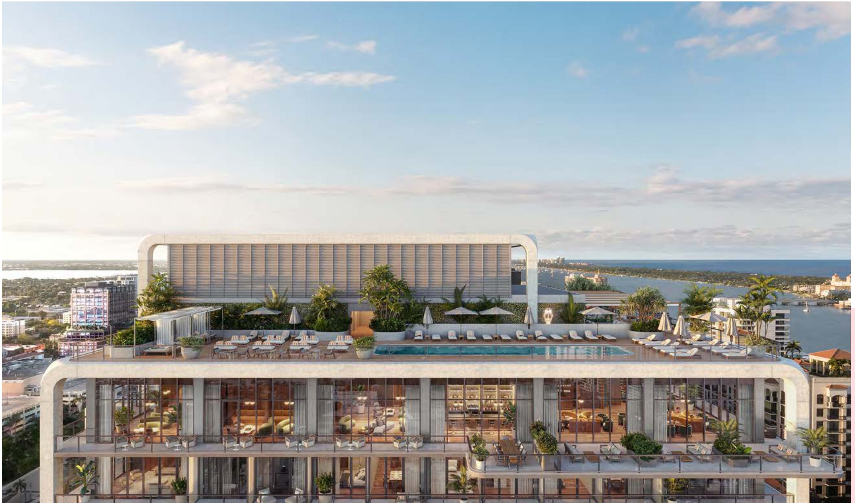
Full-Service Pool, Deck & Lounge
