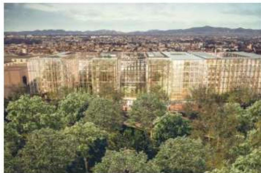
ENEL HEADQUARTERS ROME
