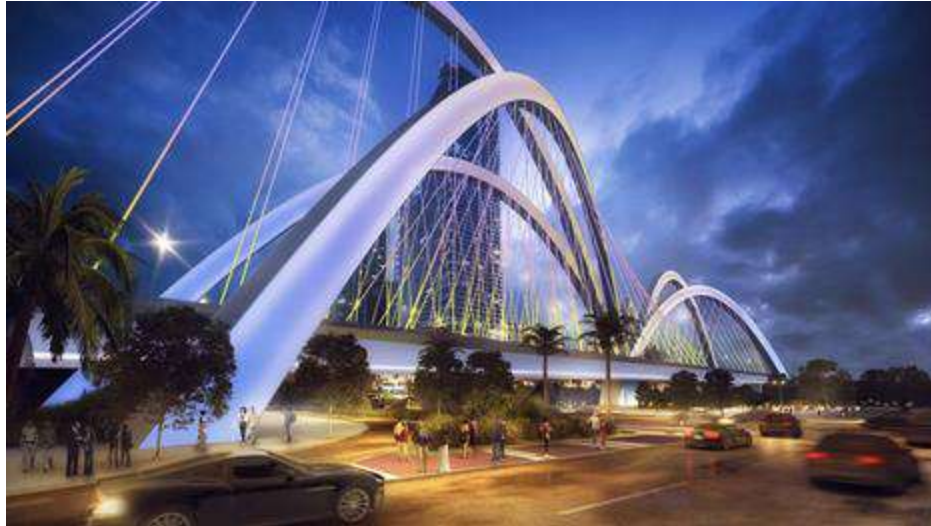
Miami Signature Bridge
