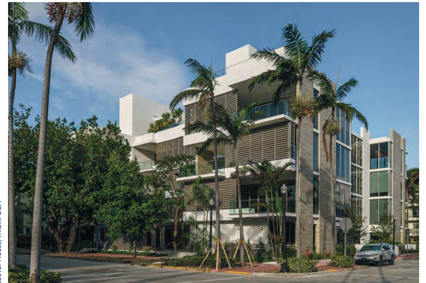
Louver House, Miami USA
