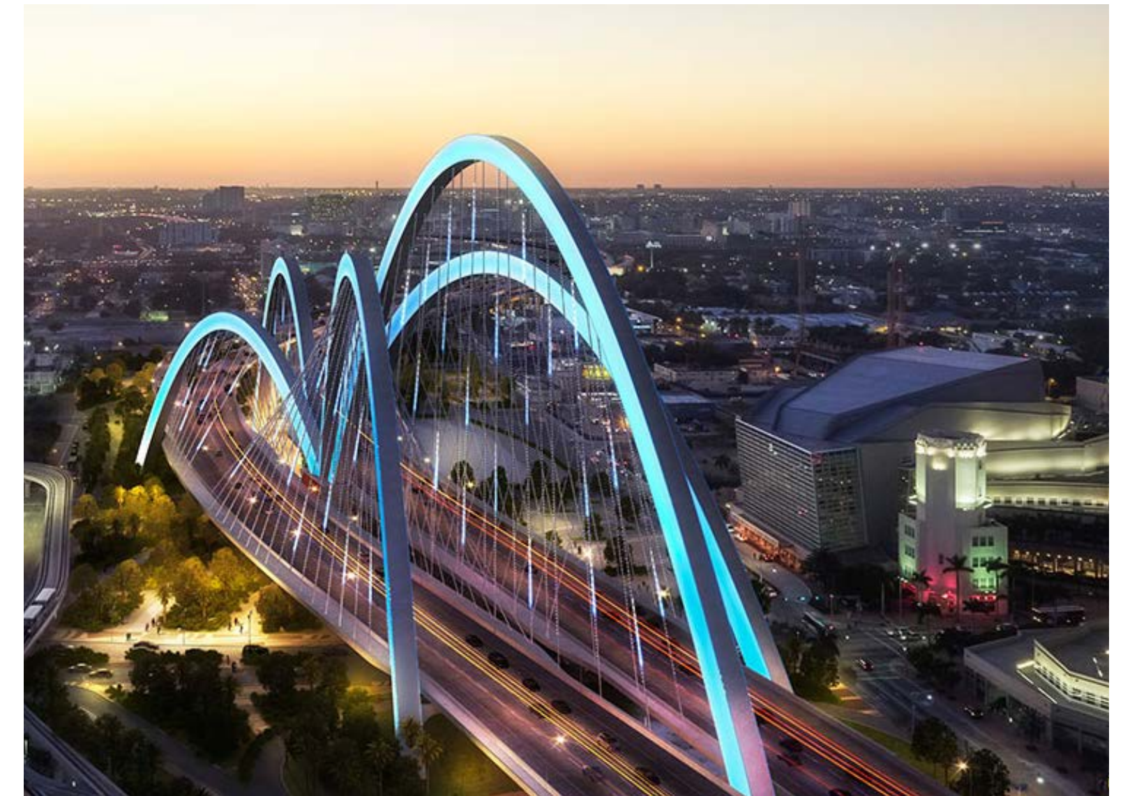
I-395 SIGNATURE BRIDGE
