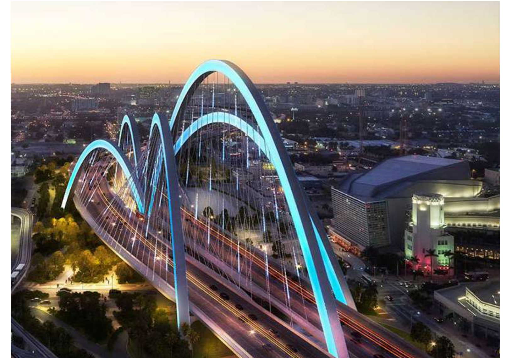
I-395 SIGNATURE BRIDGE
