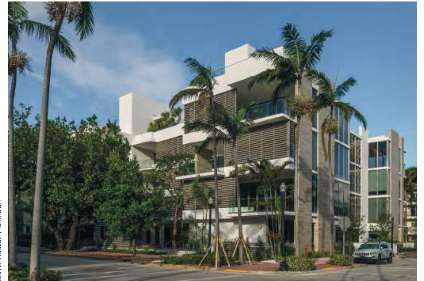
Louver House, Miami USA
