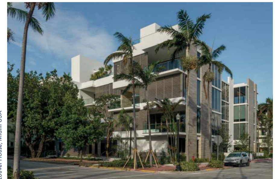
Louver House, Miami USA
