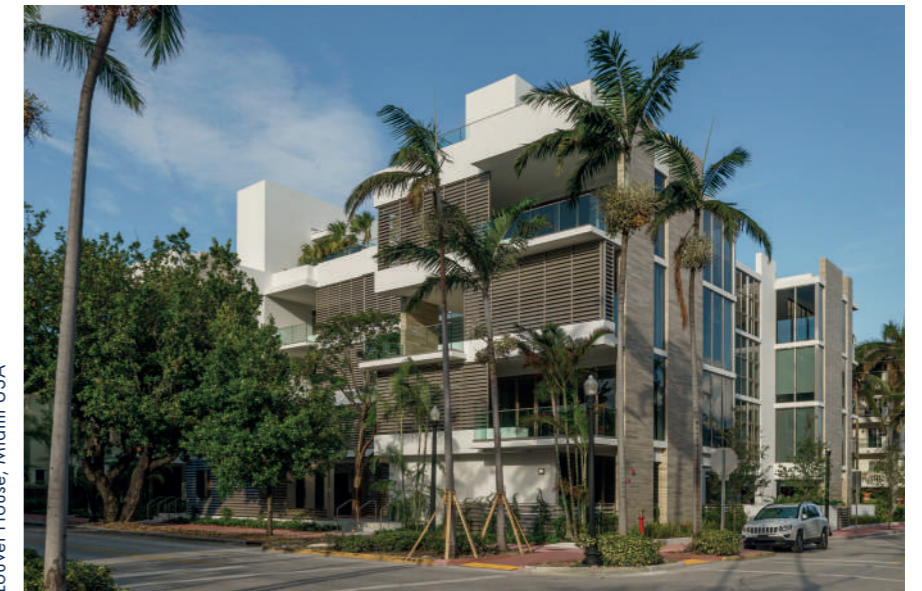
Louver House, Miami USA
